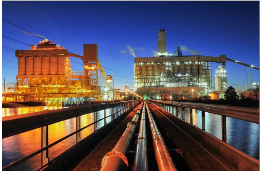
Figure 6 Cleco's 660-MWe Madison Unit 3 is a multi-fuel CFB power plant that typically burns a 80% petcoke/20% coal mix. The unit is located at the utility's Brame Energy Center, Boyce, Louisiana
