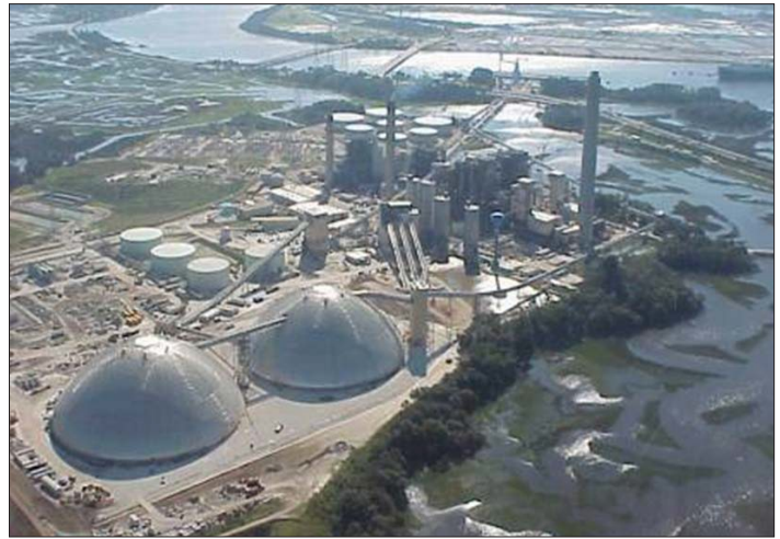
Figure 5 JEA's 600 MWe CFB power plant firing petcoke and coal at the Northside generating station in Jacksonville, Florida
