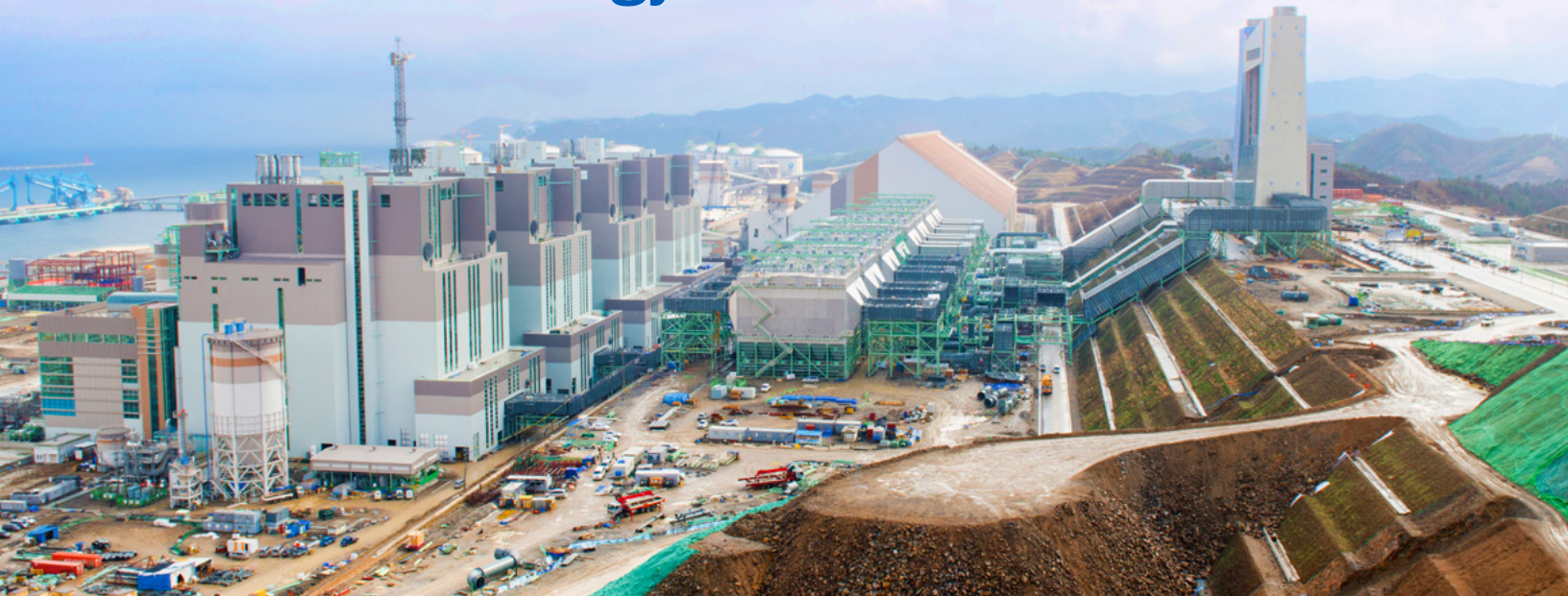
The Samcheok Green Power Plant in South Korea features 2,000 MWe of our advanced ultra supercritical CFB technology.
