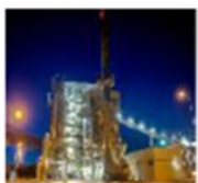
CFB and BFB boiler power plants
